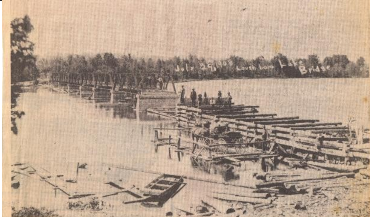
LOUGHBORO LAKE BRIDGE, BUILT 58 YEARS AGO, IS A FAR CRY FROM TODAY'S TROUBLED SPAN Lake Bottom Condition Has Caused Engineering Trouble for Frontenac County Officials
